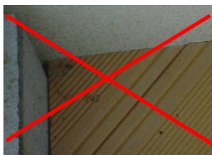
Leave a 5 mm gap between boards in width and a 15 mm between end and a wall
