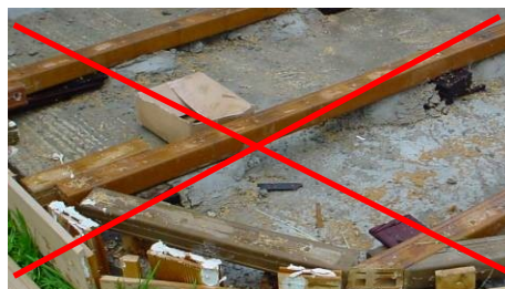
Leave a 10 mm space between ends when butting the bearers
