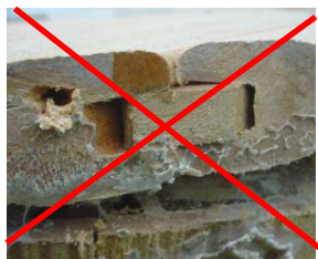
No inserts in board grooves
