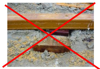
Do not steal bearers in concrete
